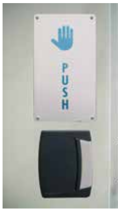
Landing door internal closing handle (only for MF Plus)
